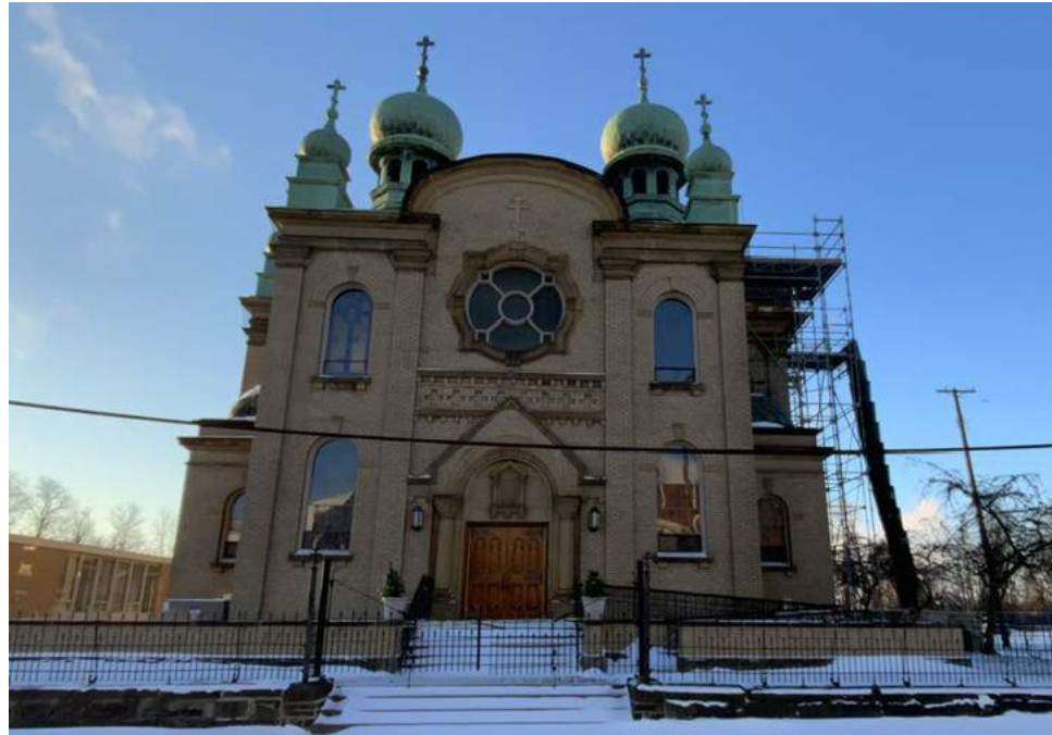
1 | VIEW OF NORTH ENTRANCE
