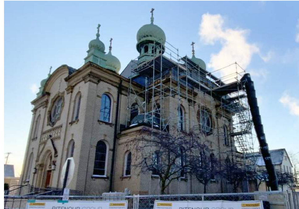
2 | VIEW OF NORTHWEST CORNER
