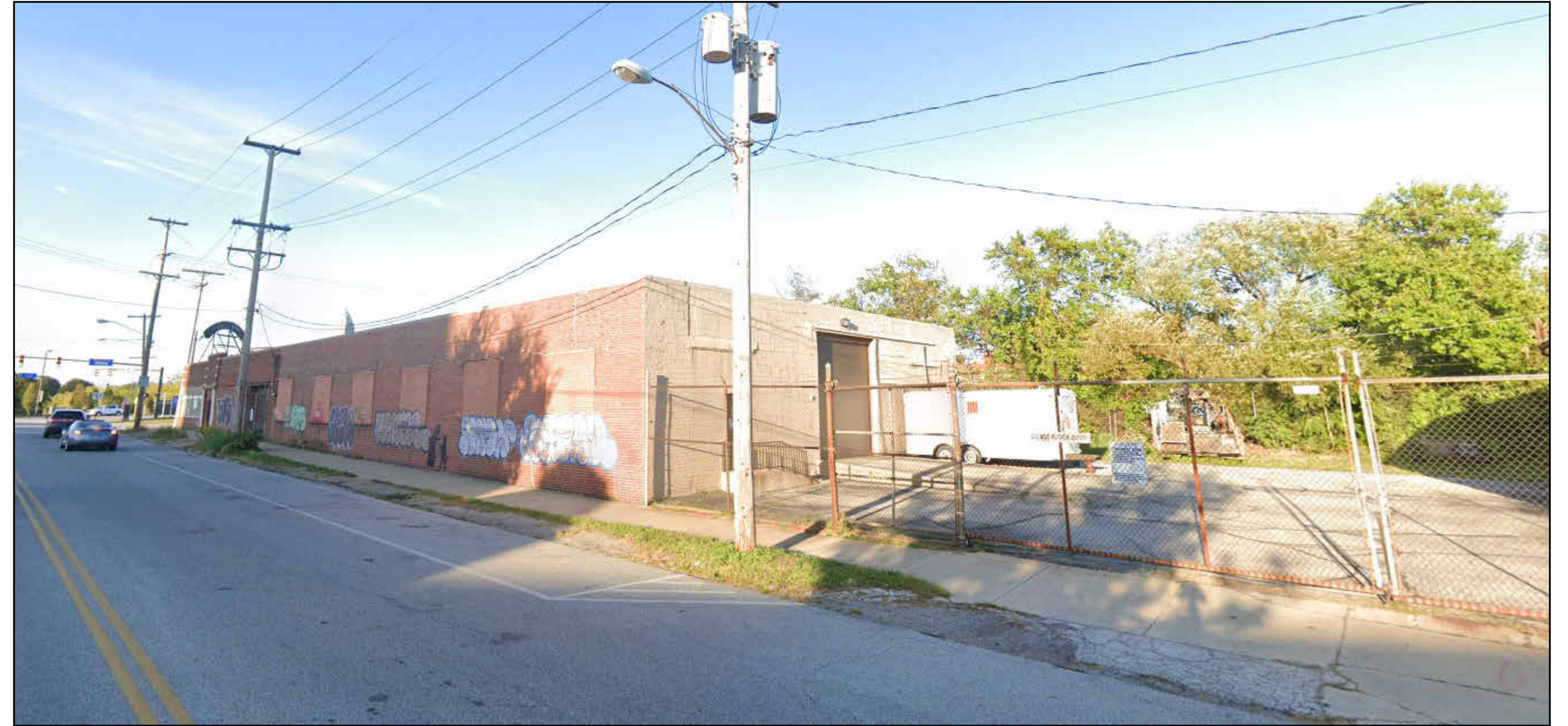
SOUTH WEST CORNER VIEW
