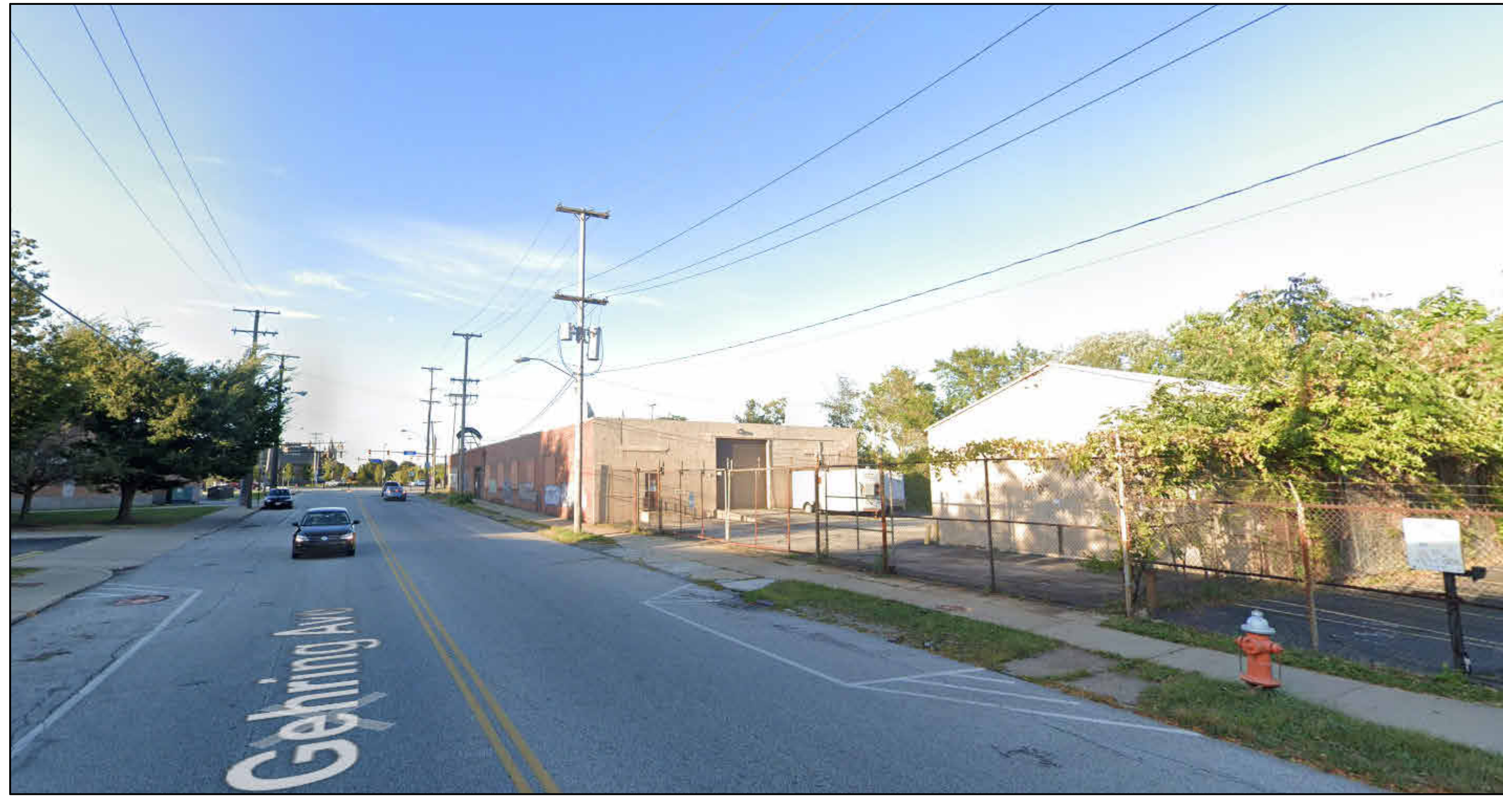
SOUTH VIEW OF SITE
